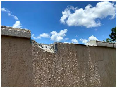
Shown below is the damage to the walls themselves that appeared more than surface-level. The corners between the walls and the pillars seem to all be fractured to varying degrees with some being surface level, and others going deeper. The mossy growth is present in many of the seemingly surface-level fractures.
